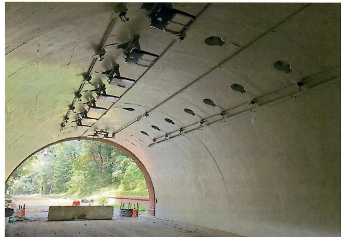
New lighting and panels installed inside the Williamsburg Tunnel.
